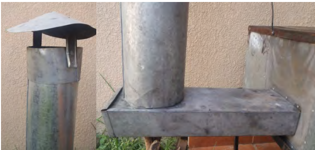
Top and bottom of the chimney pipe
